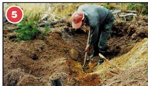
5. A conductor detected at depth may be followed along strike until it comes close to the surface, as shown here, where it can easily be dug out.
